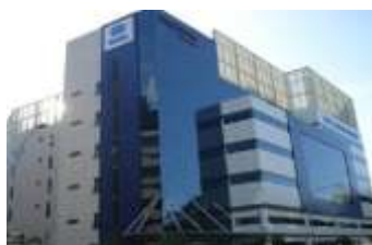
Light Industrial Buildings
