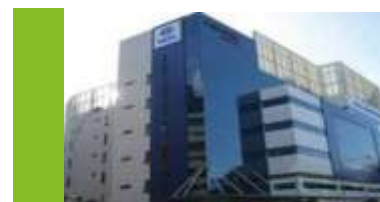
Tata Communications Exchange
